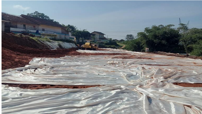
Figure 2.12 Non-woven Geotextile
